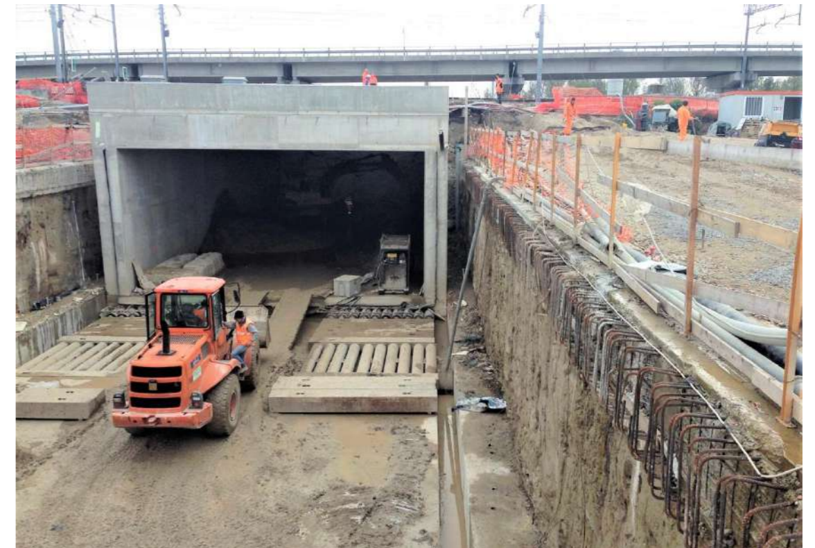
Figure 8 - Box jacking process final phases
