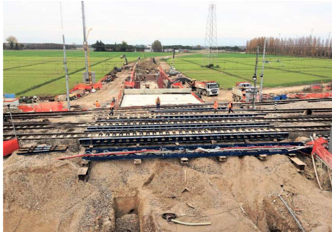
Figure 3 - Verona System Temporary Bridges installed on active tracks
