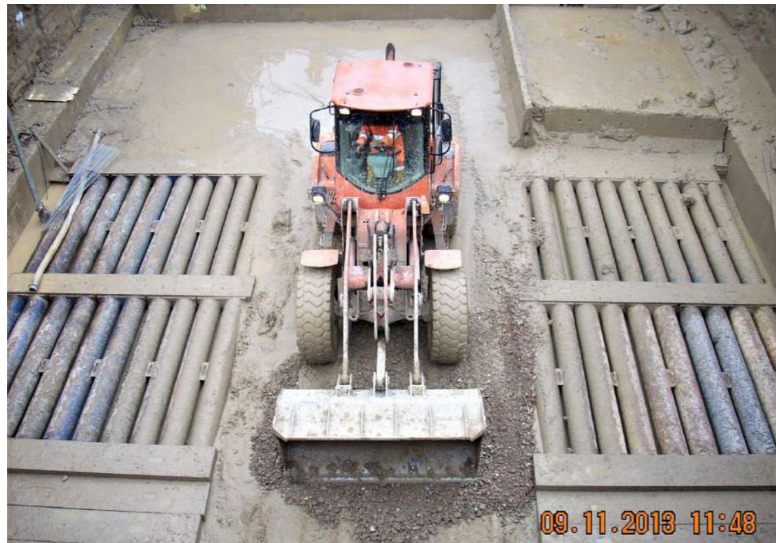
Figure 7 - View from above of the spacers of the Box Jacking system
