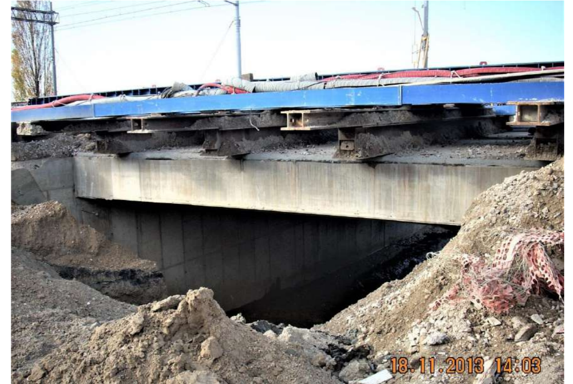
Figure 6 - Box pushed under Verona System
