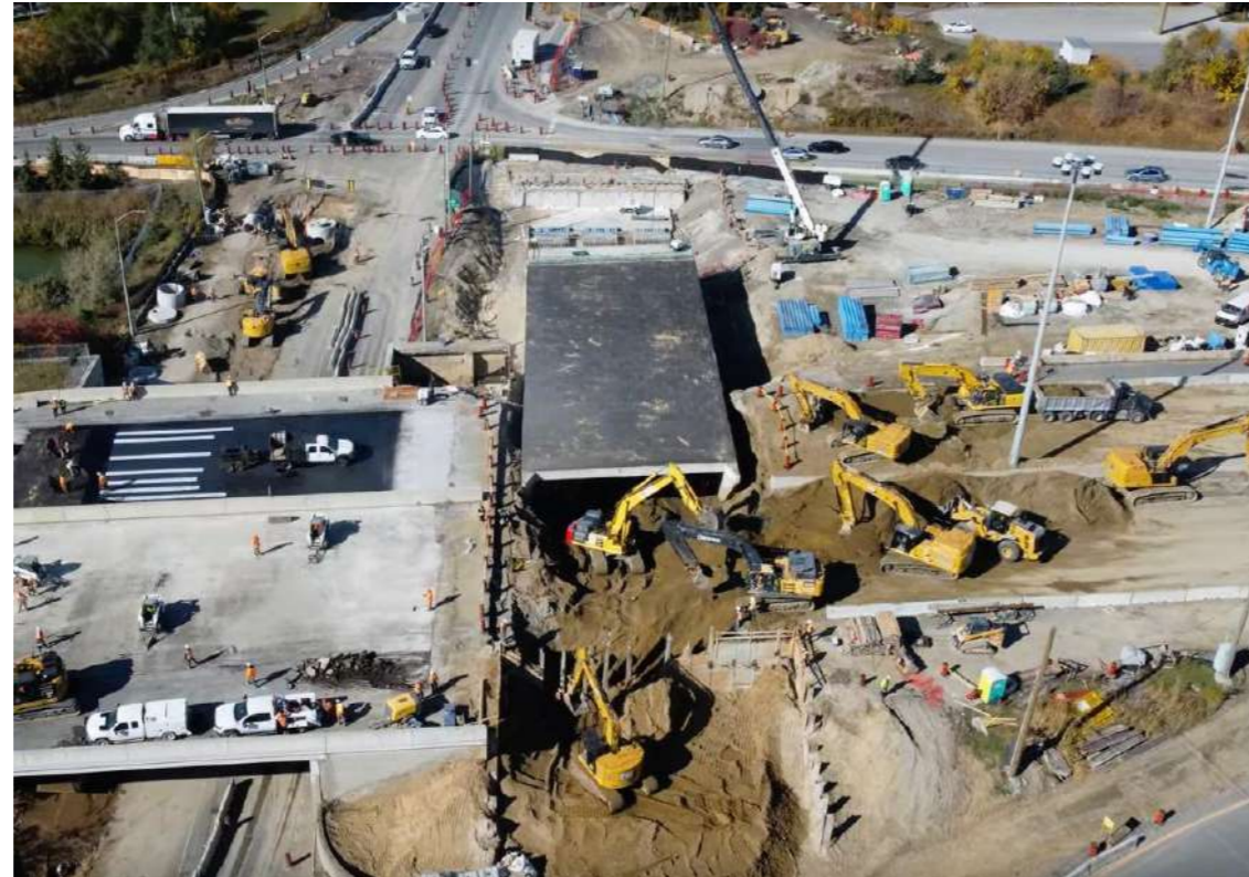
Figure 5 – Open pit box jacking and temporary road closure
