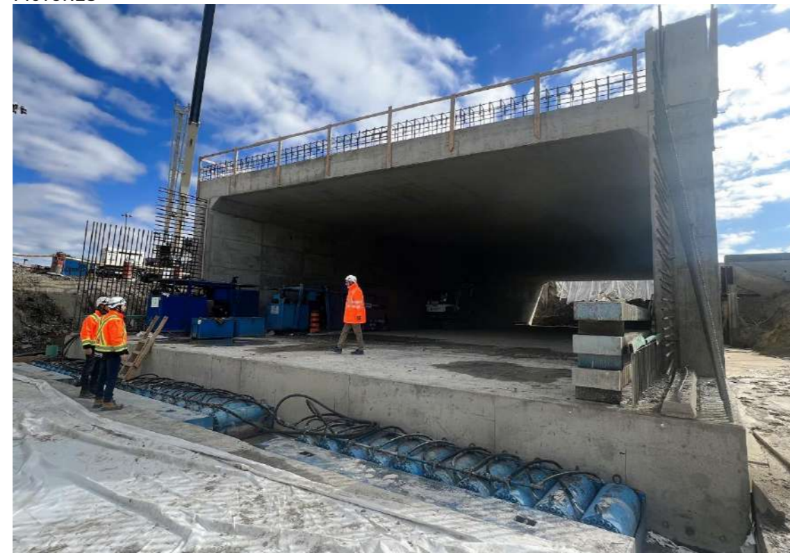
Figure 3 - Beginning of Box Jacking
