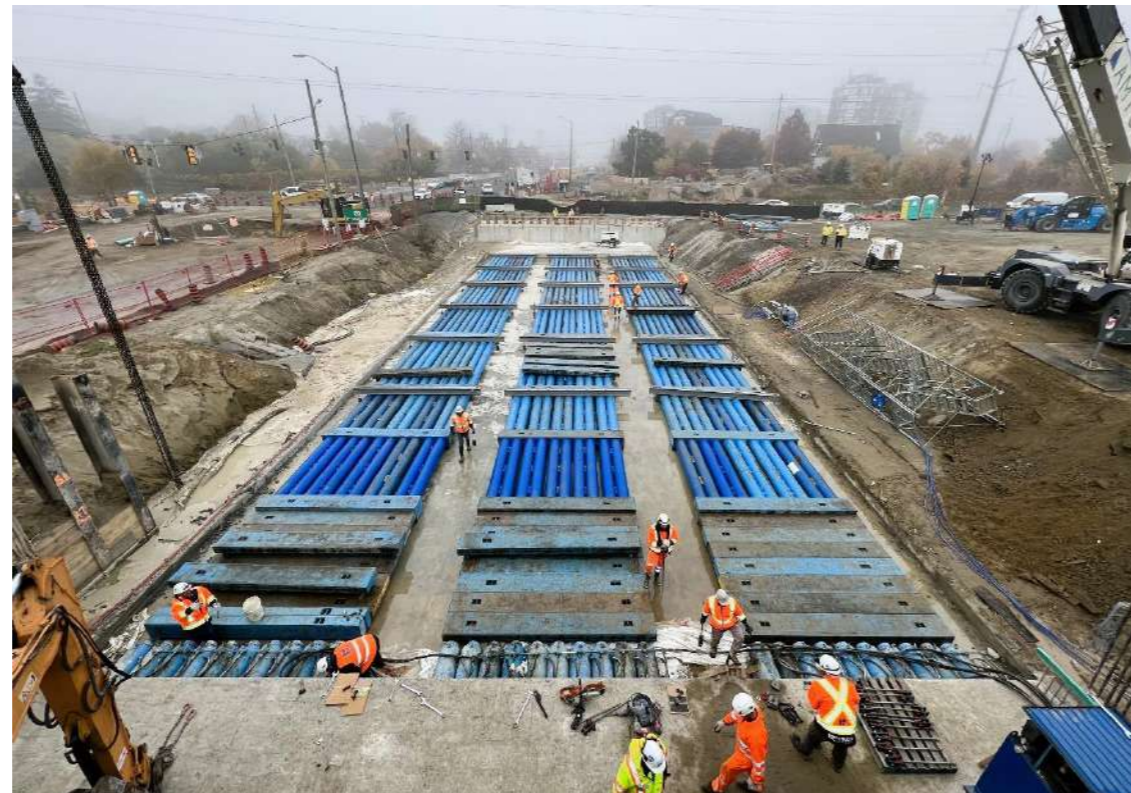
Figure 7 – Jacking columns at the end of the push
