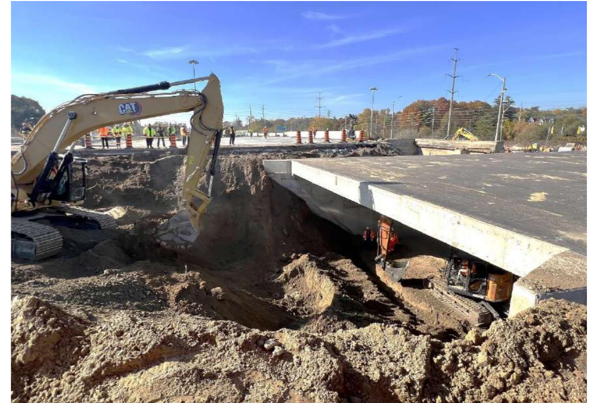
Figure 6 – Excavation from the outside
