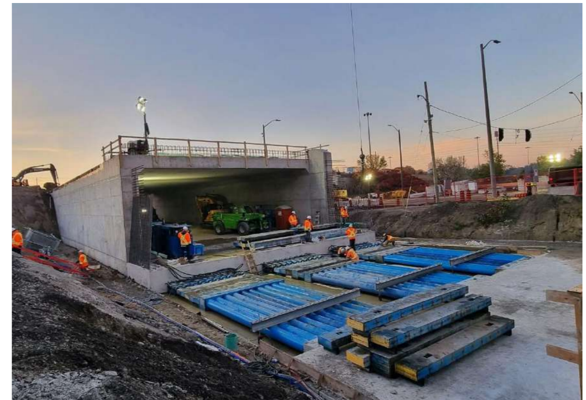
Figure 4 - Box Jacking with jacks and spacers
