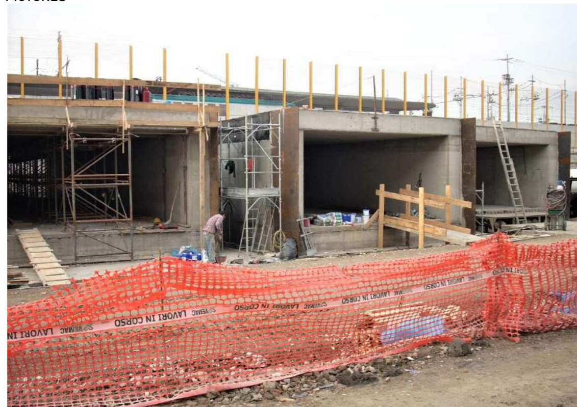
Figure 2 - Boxes In construction
