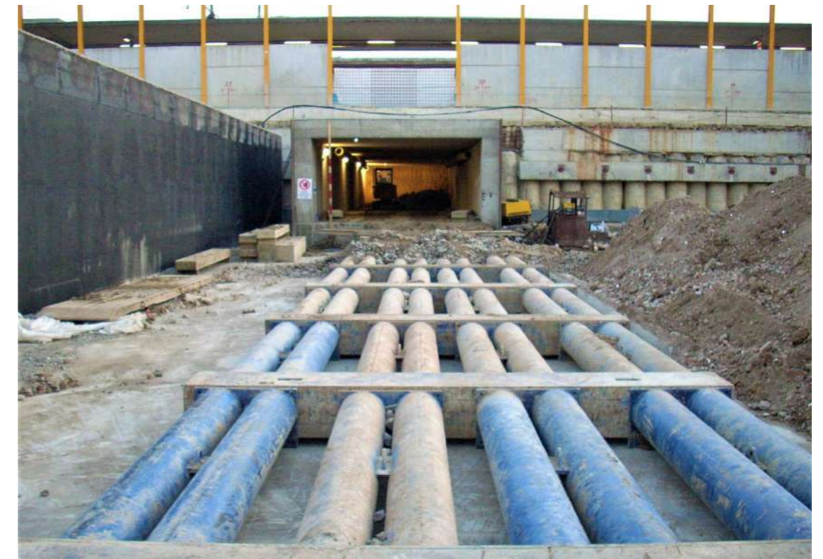
Figure 3 - Jacking of Box 1
