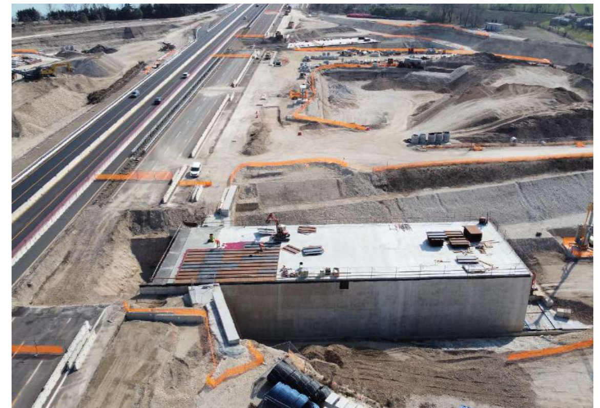
Figure 4 - View of the two boxes and Anti-drag system intallation
