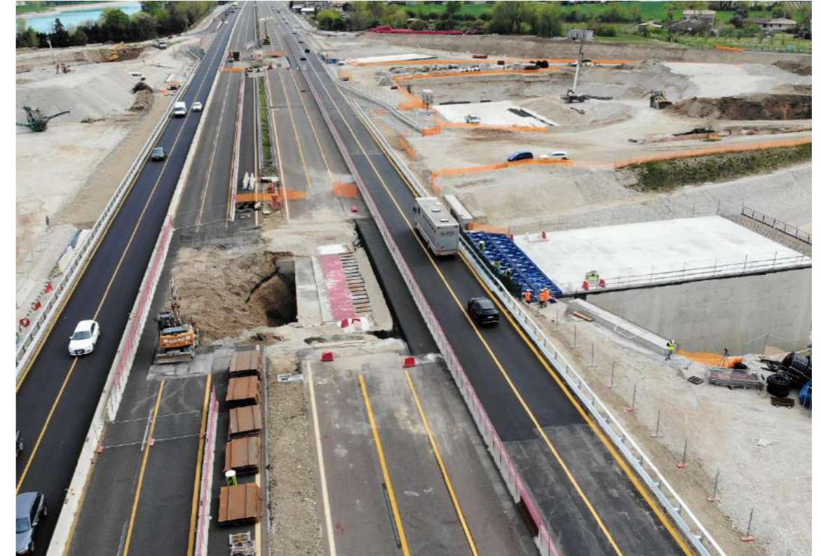
Figure 6 - Box sliding under highway with active traffic flow over Anti-drag system
