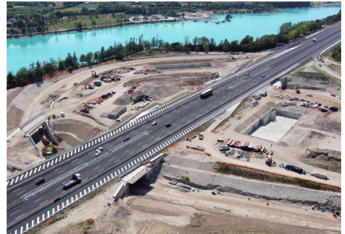
Figure 8 - Boxes jacked under highway and highway fully reconstructed
