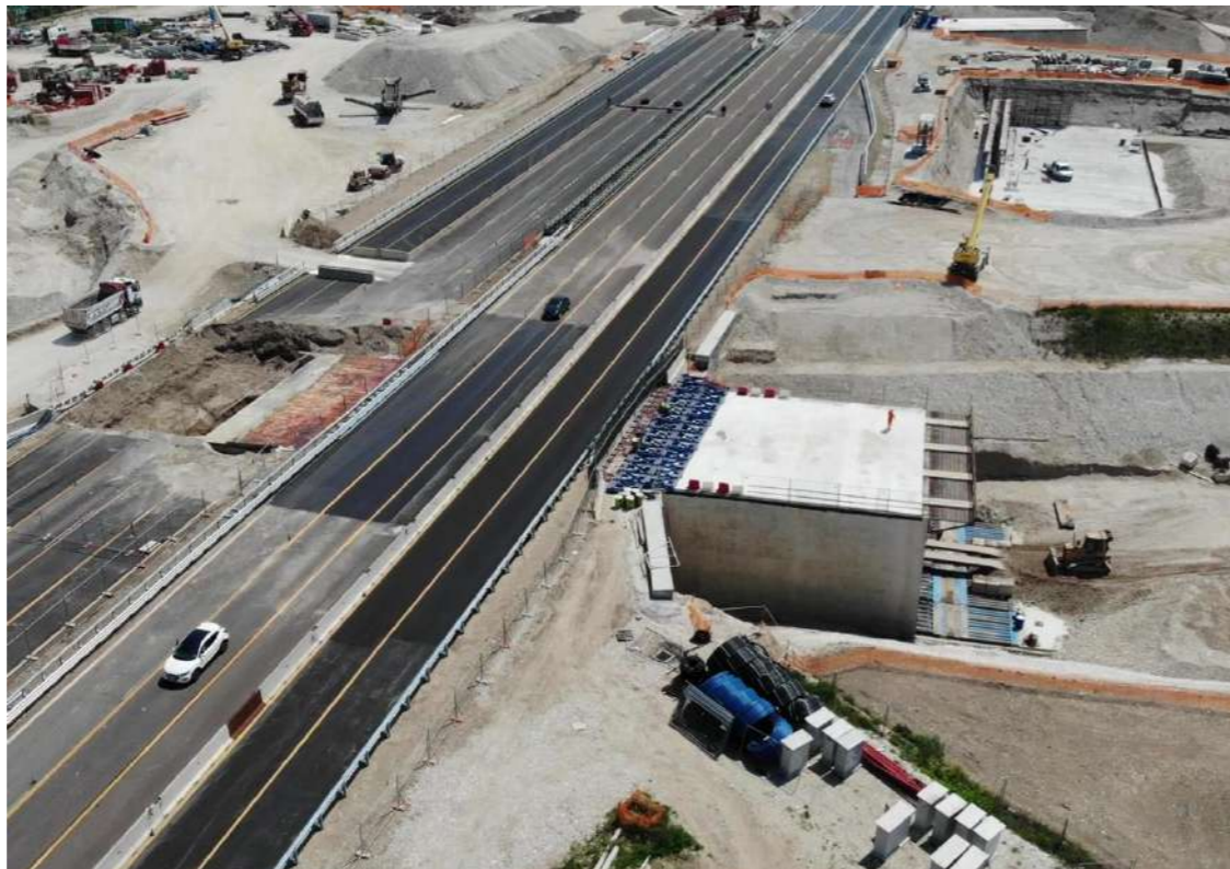
Figure 7- Double-lane reconstruction over Anti-drag system
