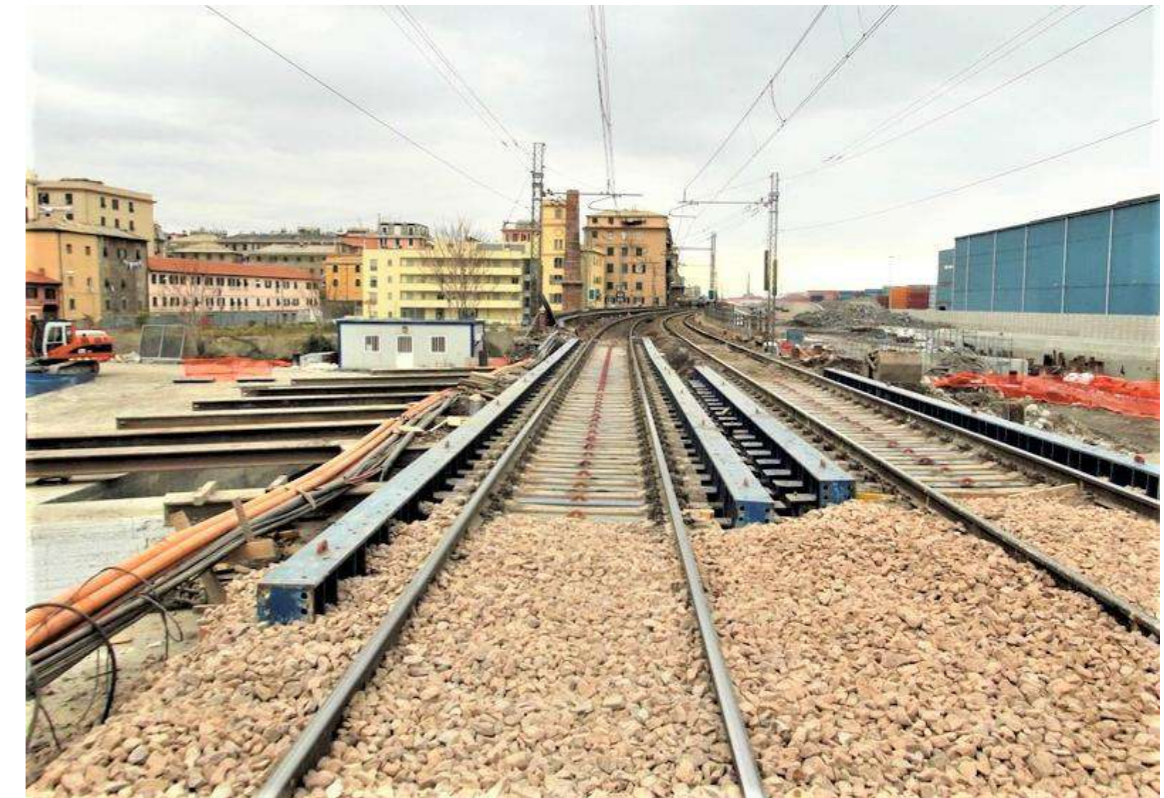
Figure 5 - Transverse beams and the Verona System
