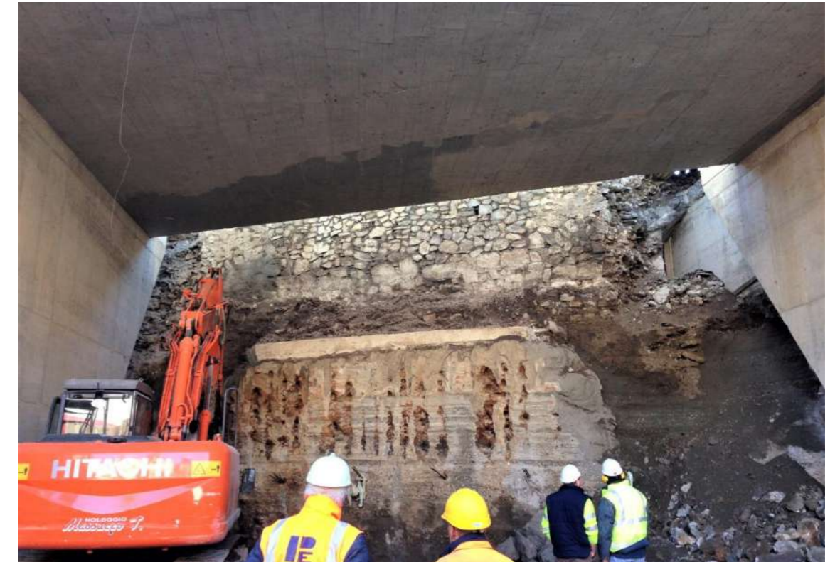
Figure 9 - Excavation from the inside
