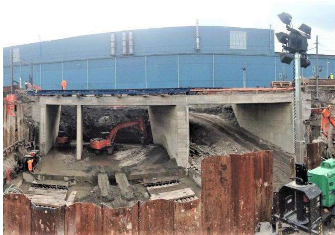
Figure 8 - Final phases of box jacking
